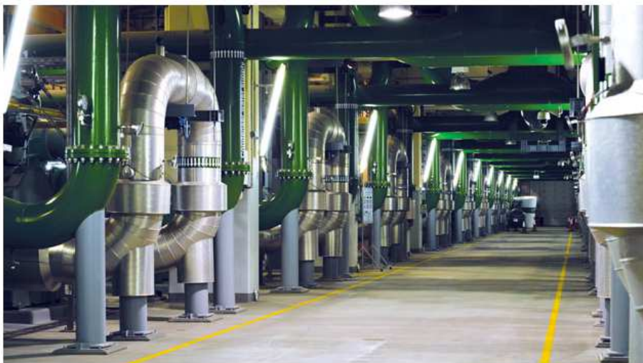
Chiller room inside the largest district cooling plan in the world, at The Pearl-Qatar. (Image courtesy Qatar Cool)
