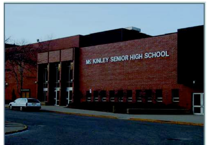
Figure 3: Test site for microturbine exhaust-driven cooling.
