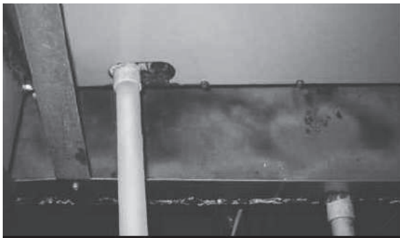
Figure4 “Slime in Drain Pan”
